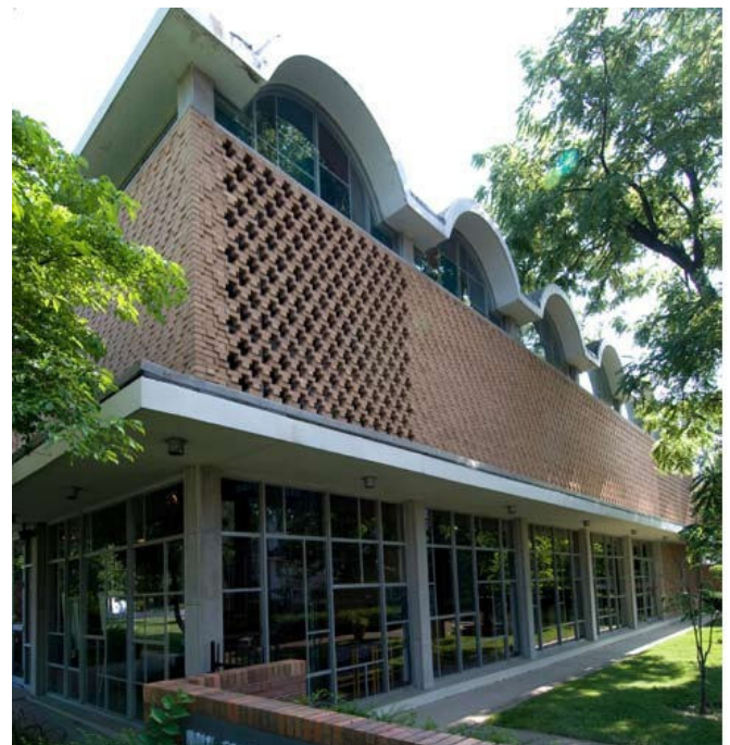
Basile Opera Center, future home of Indianapolis Opera
